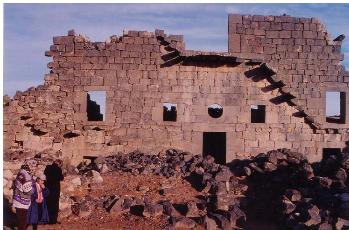
Fig. 4. Cantilevered stairways – Praetorium Umm el Jimal
